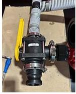
**Step 9:** Ball valve install for intake on pump, then connected to pump discharge.
